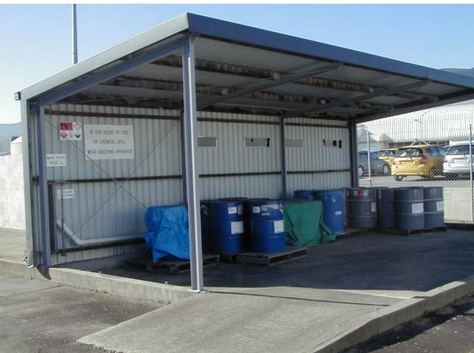
*Some good examples of HSNO compliant storage: note the forklift-friendly bund, drain valve and signage. All this class 6 and 8 product does not require a LTC in its own right*
