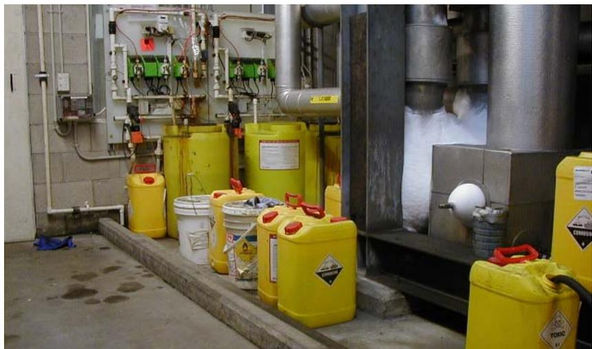
*A refrigeration site that doesn’t need a LTC because ammonia circulating internally does not trigger a LTC. However, note the drum of Class 5 and all the Class 6 and 8 scattered around the refrigeration room. Clearly a site that needs a major tidy up, but likely to be HSNO compliant, until all the Class 6-8 is caught up in a LTC process.*
